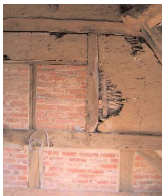
Gunnells in progress
