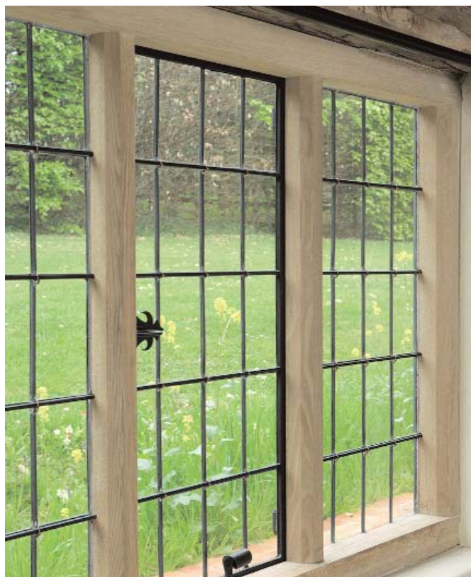
The modern glass in the windows were replaced and re-leaded using hand-made glass
